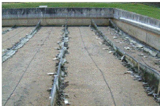
AquaMats® in polishing cell with later view of surface biofilm and invertebrate colonization on an AquaMat after 6 weeks in wastewater lagoon. When combined with ADS fine bubble diffusion and BactaPur's formulations, AquaMats® support the animal (as opposed to the plant or algal) side of the biological food chain and convert vast quantities of organic waste into aquatic animal life!
