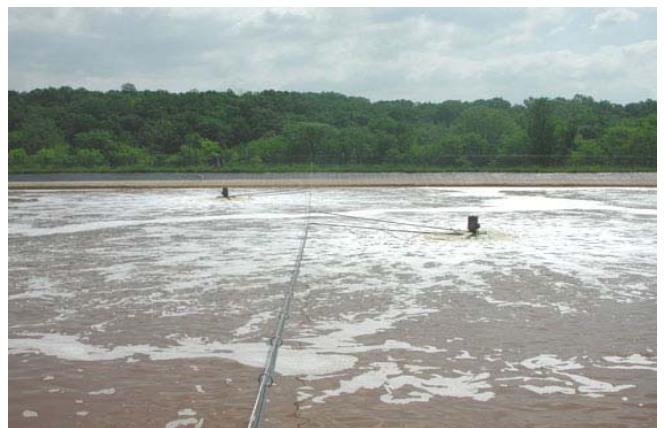
Primary Cell (Before) Surface Aerators Only
